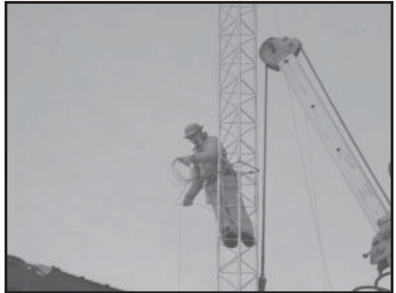
Brother Justin volunteers 60 feet above Galena soil working to place a transmitter cable for station KIYU, a listener supported public radio station operating on 910 AM.
